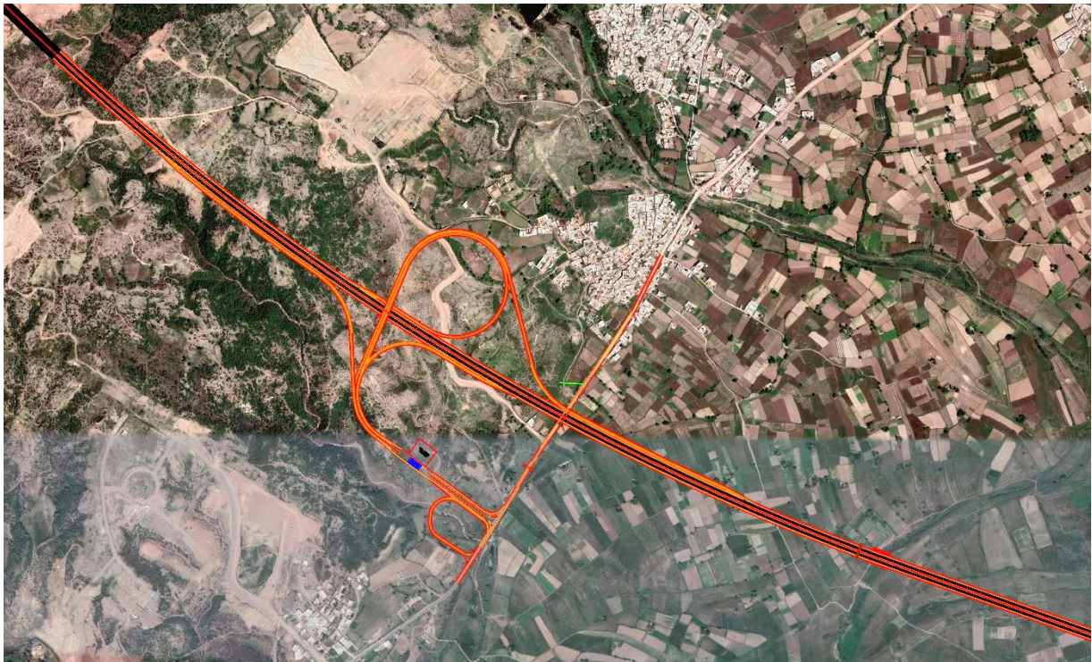
Partial Clover leaf interchange at Adiala Road crossing (Future)
